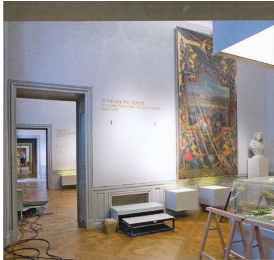
Figure 1 – Solid surface light boxes were installed on the lower wall to accomplish 3 main objectives; illuminate the paintings; offer information about the exhibits via backlit inscriptions; and serve to prevent the public from getting too close to the priceless works of art.
