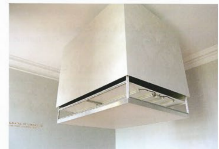
Figure 7A – Large chandeliers made of solid surface engraved in the same patterns as the wall panels hang from each of the rooms. On average they weigh about 1,100 lbs.
