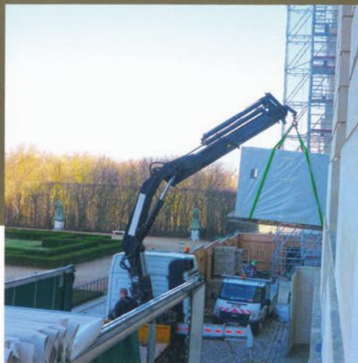
Figure 8 – The immense project used 16,000 sq. ft. of solid surface, which had to be hoisted into the building using a crane system. When completed, the solid surface portion of the project took more than 12,000 man-hours.
