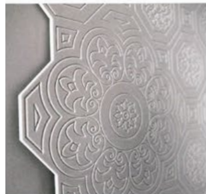
Figure 3 – Installing panels with such intricate and exact patterning without damaging the engraving was a bit of a challenge. CREA Diffusion overcame that by cutting the panels into sections with “puzzle-shaped” edges.
